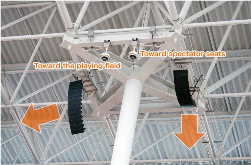
Main stand speakers oriented toward the playing field (left) and toward spectator seats (right)
