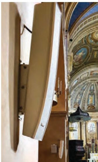
TOA SR-H2S column speakers are fixed either side of the nave
