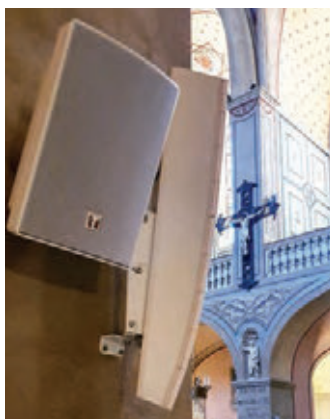
TOA SR-H2S column speakers are flanked by BS-1030 in-wall speakers
